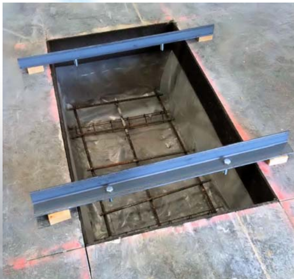
ATW, VTW & AIT-238 Isolation Pad Installation Preparation
